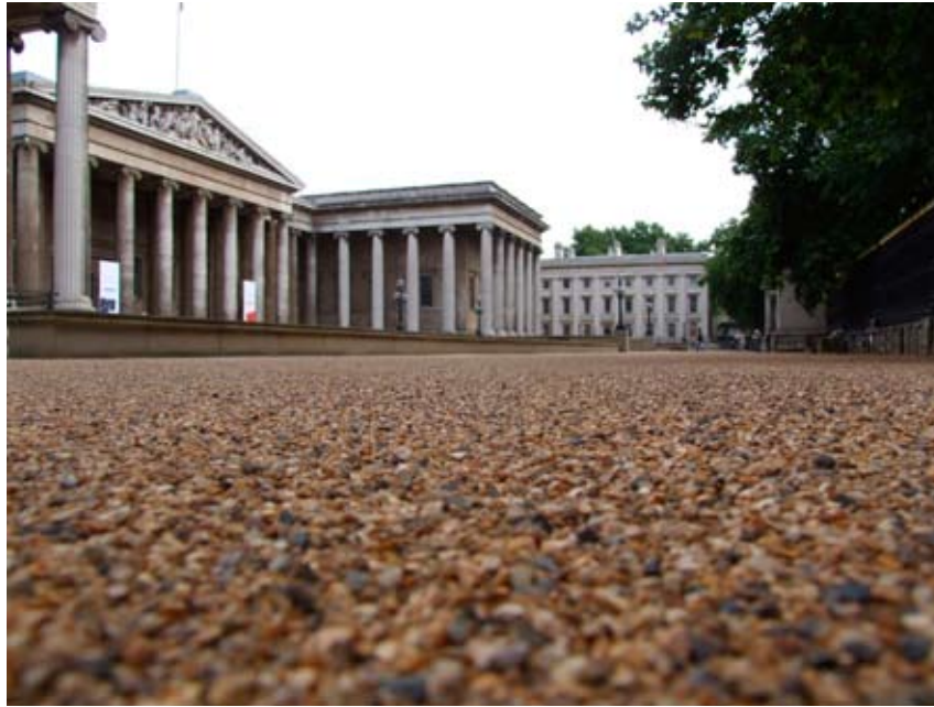
The grounds of the British Museum have been surfaced with Addagrip's Addastone; an attractive and hardwearing resin bound surfacing.
